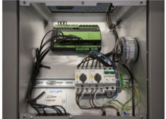
All electrical and control equipment is collected inside a special enclosure in the centred section of the air handling unit.
